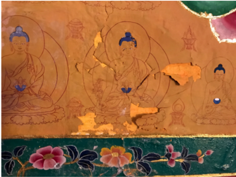
These wall paintings have been repainted many times. The paint continues to peel because the monastery walls are wet outside and the water seeps through the wall to the inside, where it damages the wall paintings.
